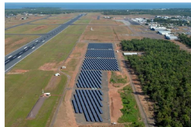
Figure 9-2: Darwin Airport – 4MW Solar Farm
