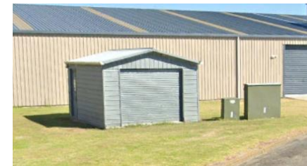
Figure 7-6: Emergency Generator Building
